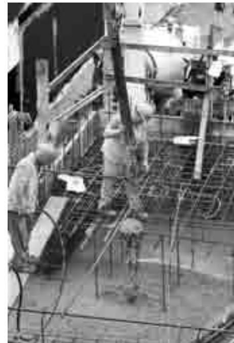
Workers direct cement through rebar as the roof is poured for the addition to the Charles L. and Rose Sweeney Melenzyer Pavilion which will house Monongahela Valley Hospital's new Image Guided Radiation Therapy unit.
