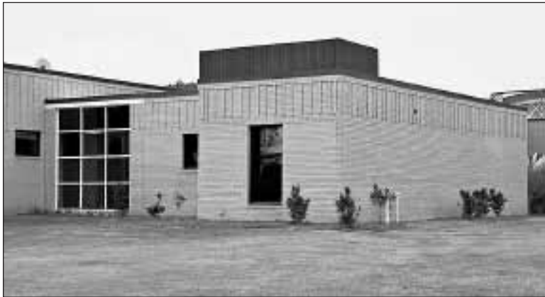
ModSpace's Nash General Hospital Modular Healthcare Construction Project in Rocky Mount, NC.
